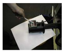
5. Dismantle new pump switchboard cover. Push the cable through the bushing and fasten it.
